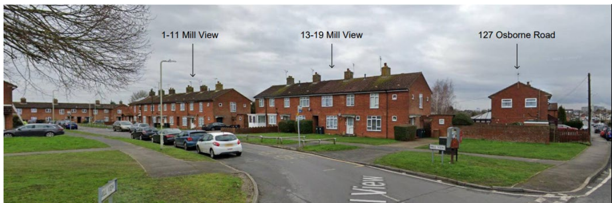
Figure 4 - Previous dwellings (now demolished)
